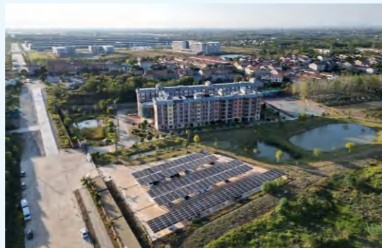
Parking Lot Photovoltaic Carport of GEM Wuhan Park
