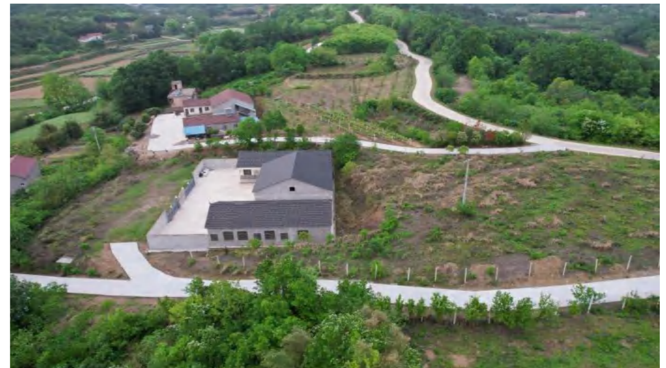
Roads in Jinghe Village under the Construction of GEM Assistance Project
