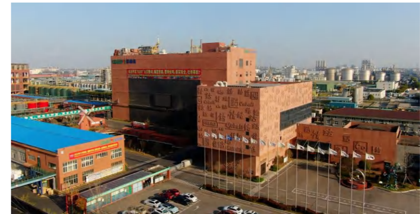
Safety and Environmental Protection Square construction at the site of the Taixing Park fire
