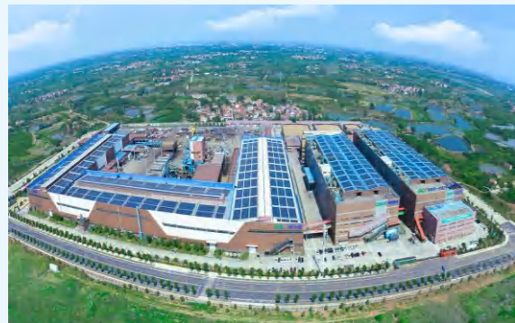
Roof Photovoltaics in the Factory of GEM Wuhan Park
